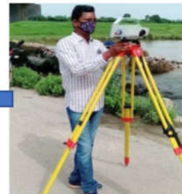
Establishment of Control Points
